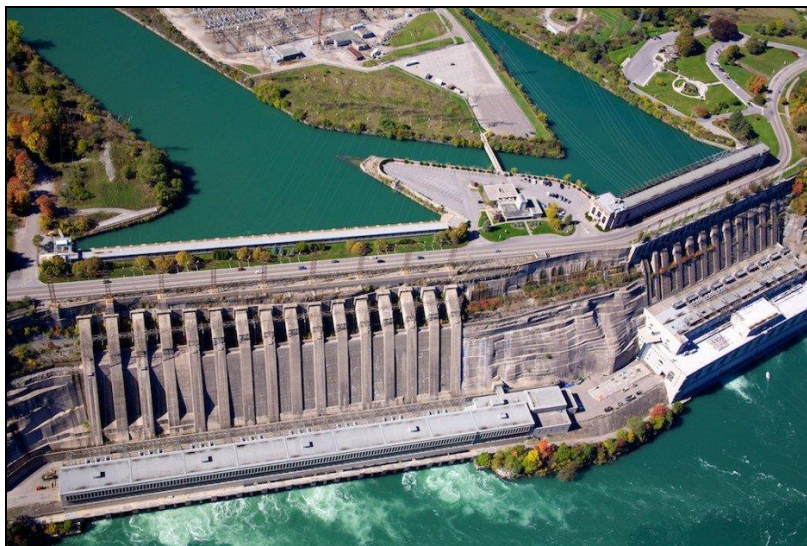
This is the Adam Beck Generating Station on the Canadian side of Niagara. The section on the right was built in 1922 and that on the left in 1952.
